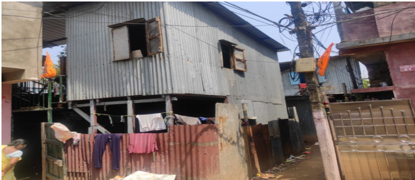
Figure 1: Displays the housing condition.
